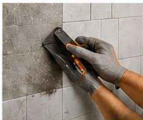
MASONRY & TILE WORK
