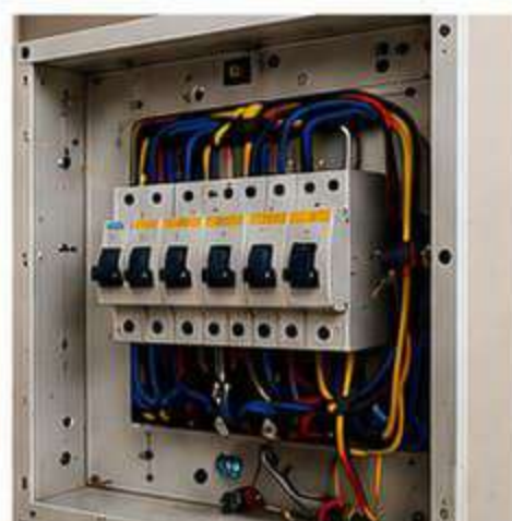
DB INSTALLATION & UPGRADES
