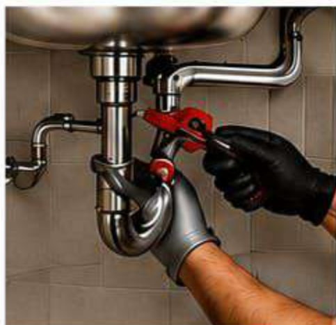
PIPE INSTALLATION & REPAIR
