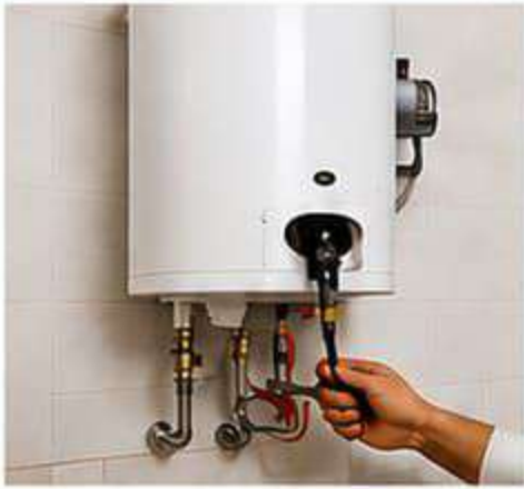
WATER HEATER INSTALLATION
